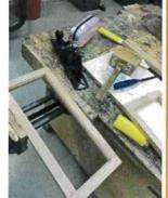
Router both frames and perfect corners and apply plywood back - A vice, bevel edged chisel, sharp pencil, tri square, 12mm Router bit, T5 Trend Router, mallet, 8 x G-cramps, PVA, scrap wood
